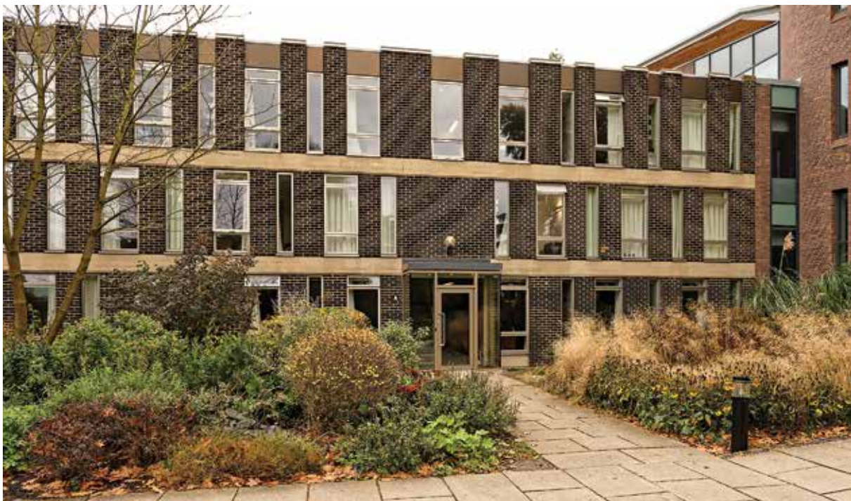
A Staircase now has an inconspicuous glazed entrance porch, which will reduce heat losses
